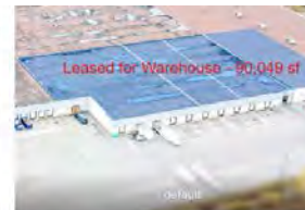
Warehouse Units C, D, E, F
