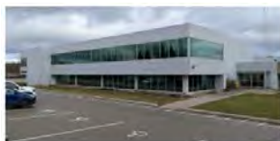
Office Units Block J, H, 2nd Floor, A1, total of four spaces.
